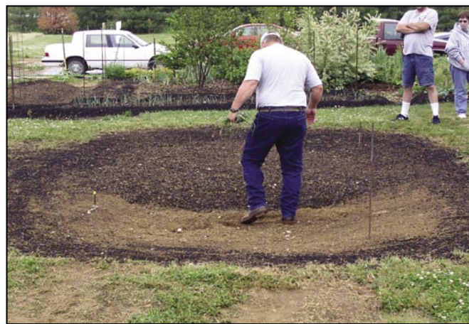
During this rain garden installation the area was over-excavated in sandy subsoil and backfilled with a soil amended with compost to increase organic matter content.
