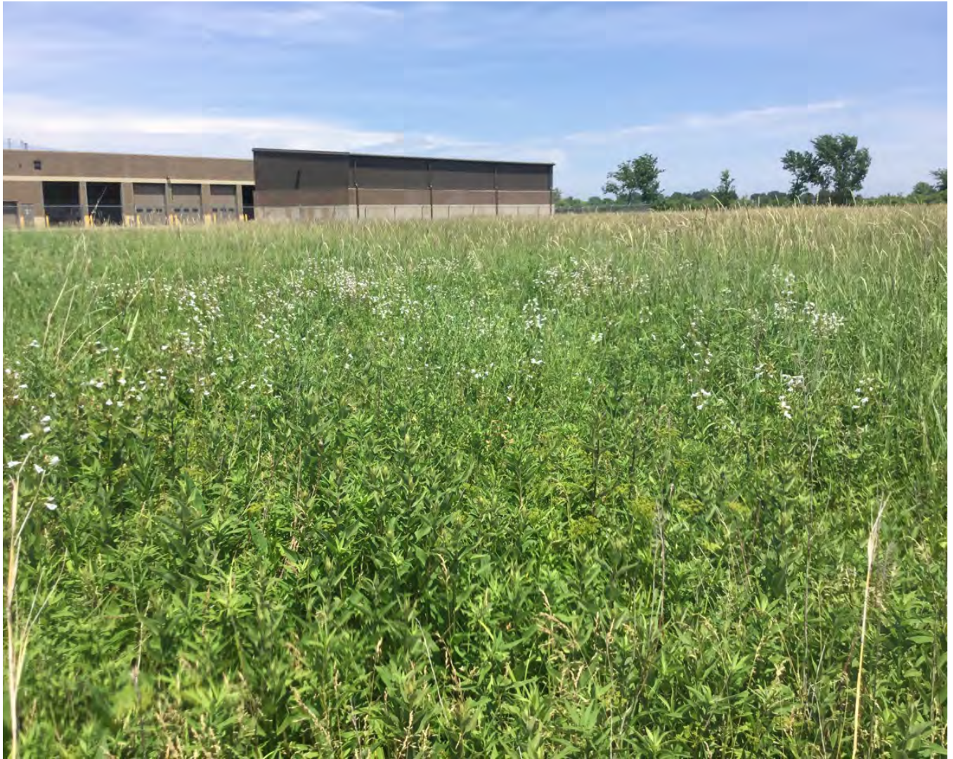
Sewage treatment building, northeast section of Iowa City Kickers Soccer Park
