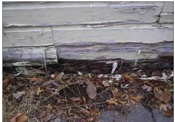
Peeling Paint, Wood at bottom is rotting
