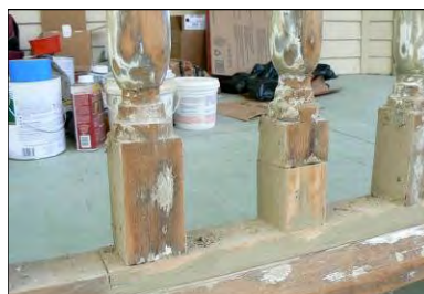
Small decay holes filled with epoxy, larger ones replaced with new wood
