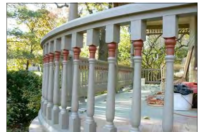
Original balusters are repaired and repainted retaining the original material and integrity
