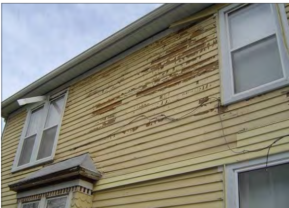
Peeling Paint, Wood likely in good condition
