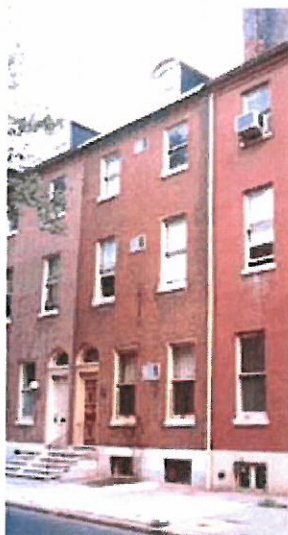
Historic building material destroyed by through-the-wall air-conditioners.
