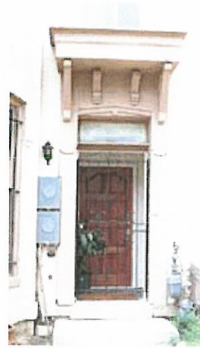
Inappropriate installation of new meters on primary elevation.
