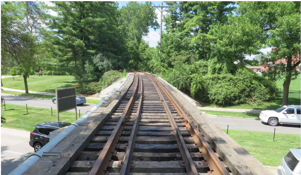
Figure 2-3: Curvature and Grade on the CRANDIC Corridor Right-of-Way at Iowa Avenue in Iowa City
