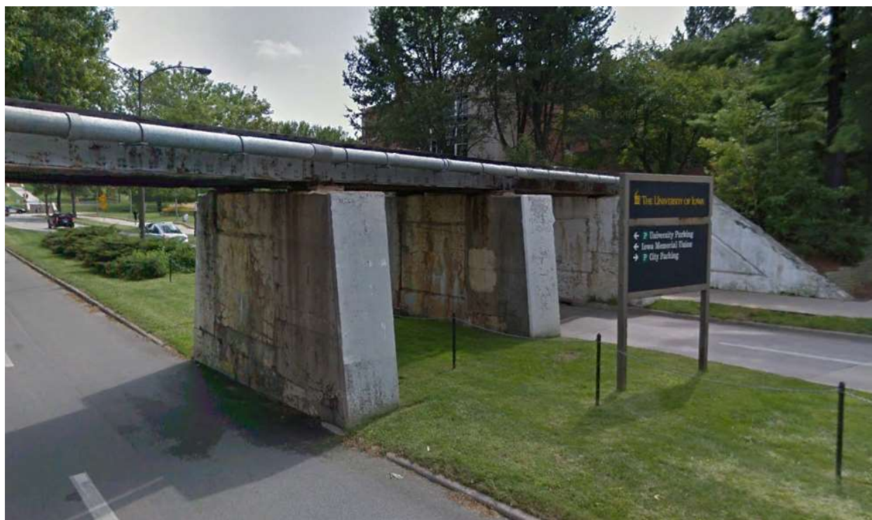
Figure 5-3: Open-Deck Railroad Bridge in CRANDIC Corridor Right-of-Way at Iowa Avenue in Iowa City
