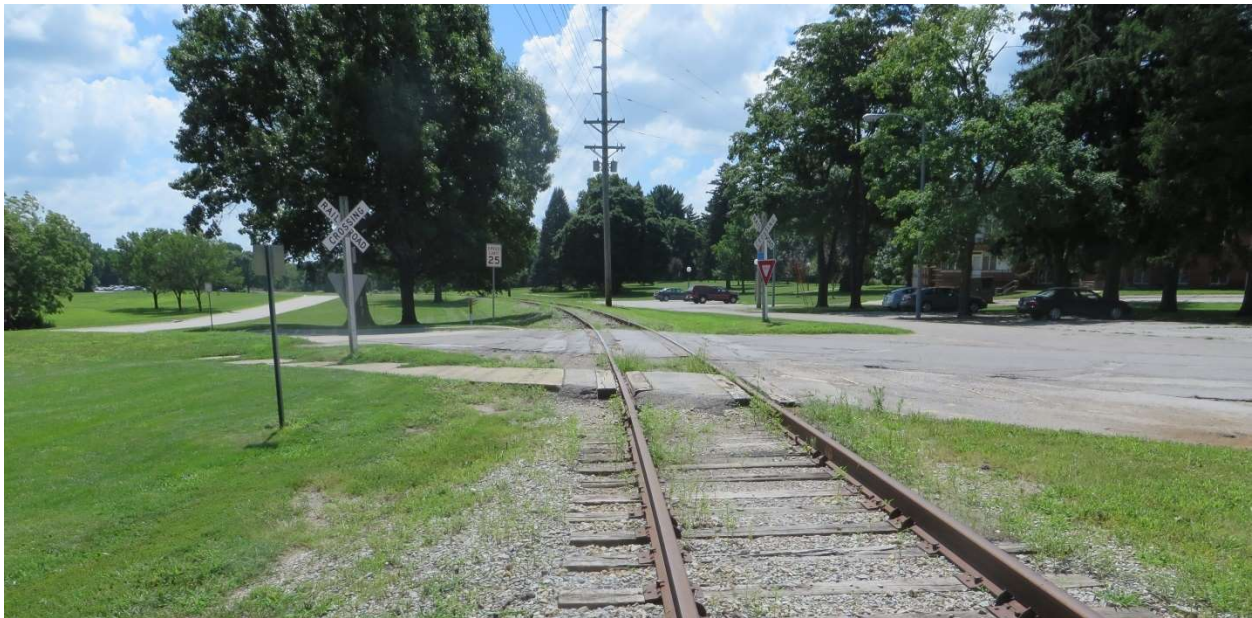
Figure 2-8: Typical CRANDIC Corridor Passive Grade Crossing at Old Hospital Road in Oakdale
