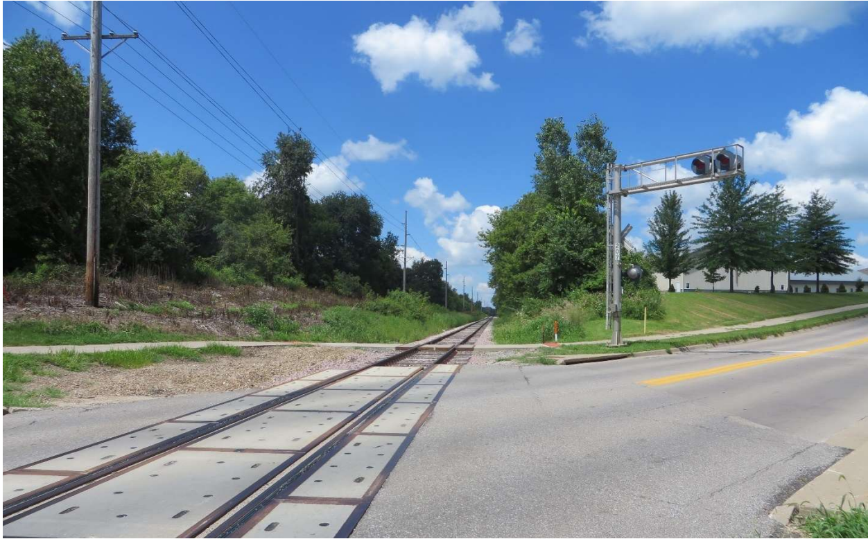
Figure 2-7: Typical CRANDIC Corridor Active Grade Crossing at 12 th Avenue in Coralville
