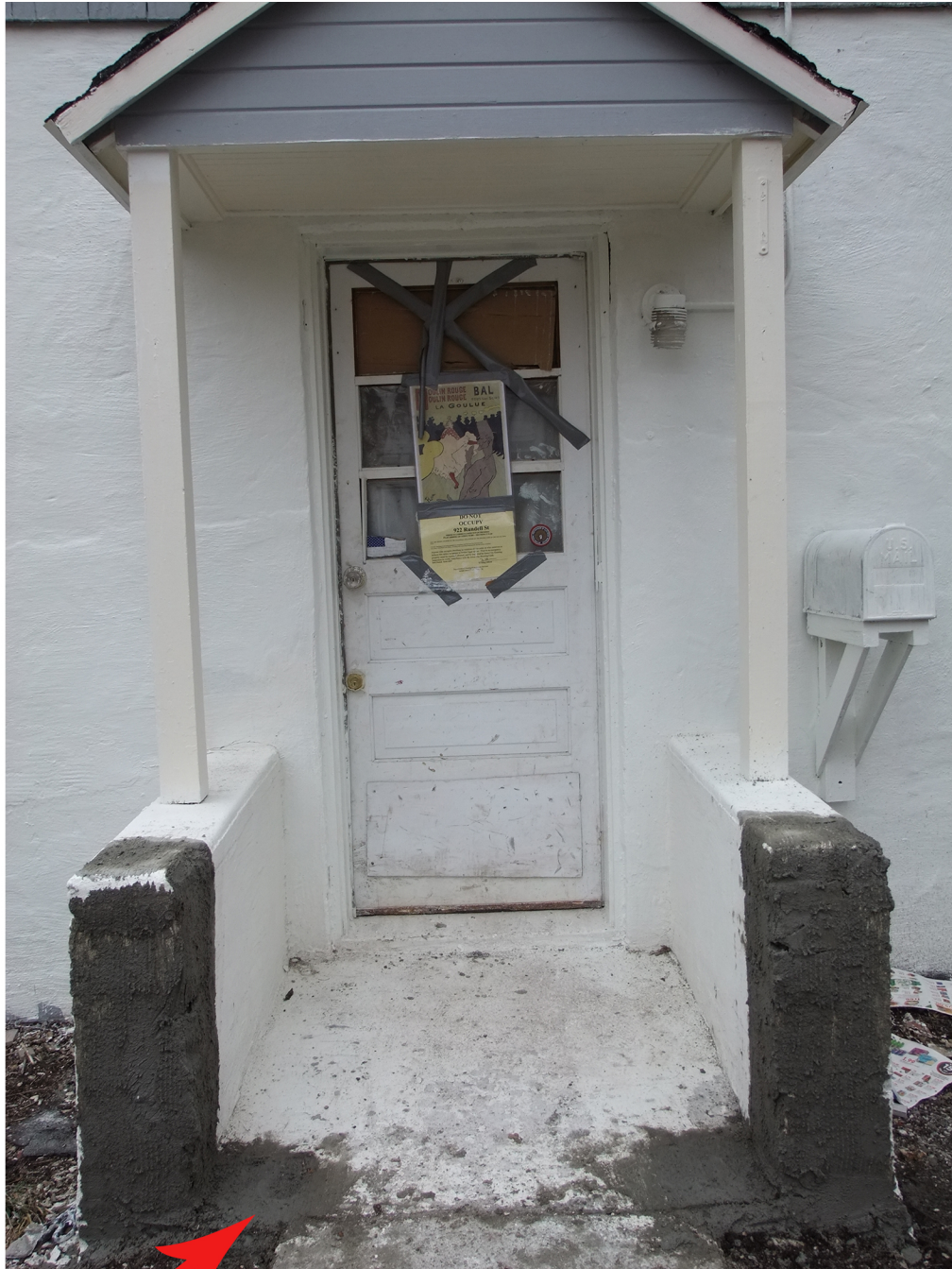
Current situation: floor slab shows where the wall used to return. Stucco coating a first scratch coat stage (unfinished)
