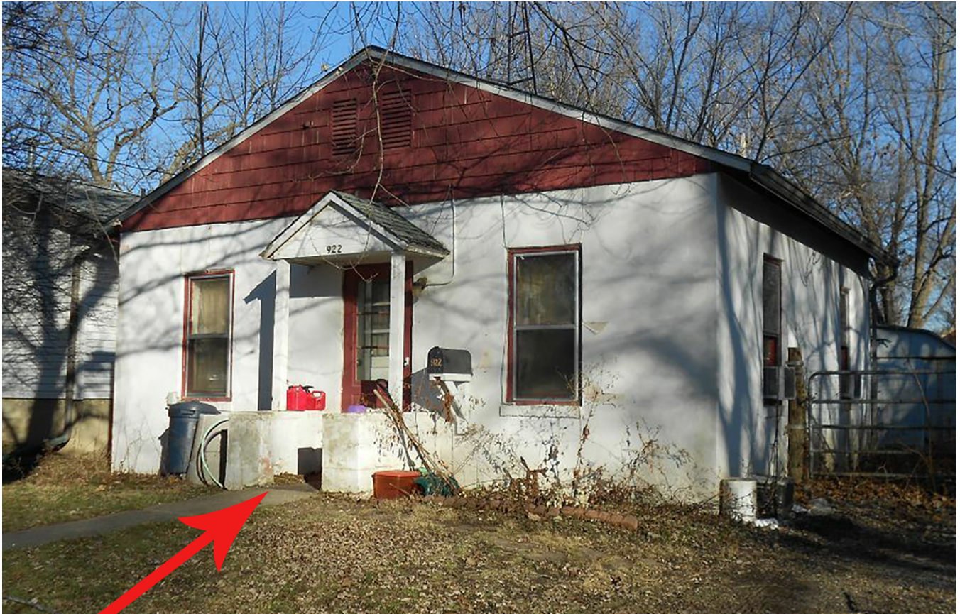
Image of front entry porch prior to work showing corner returns at west wall
