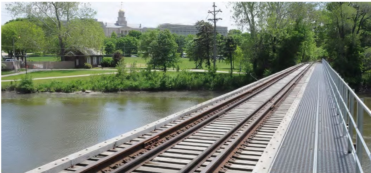
Figure 9: Iowa River Bridge in Iowa City
