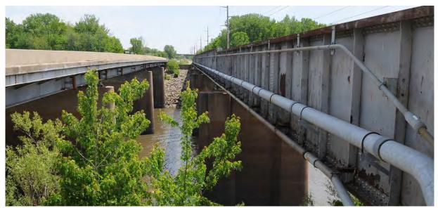
Figure 12. Fiber Optic and Utility Infrastructure in the CRANDIC Corridor near Mid-River
