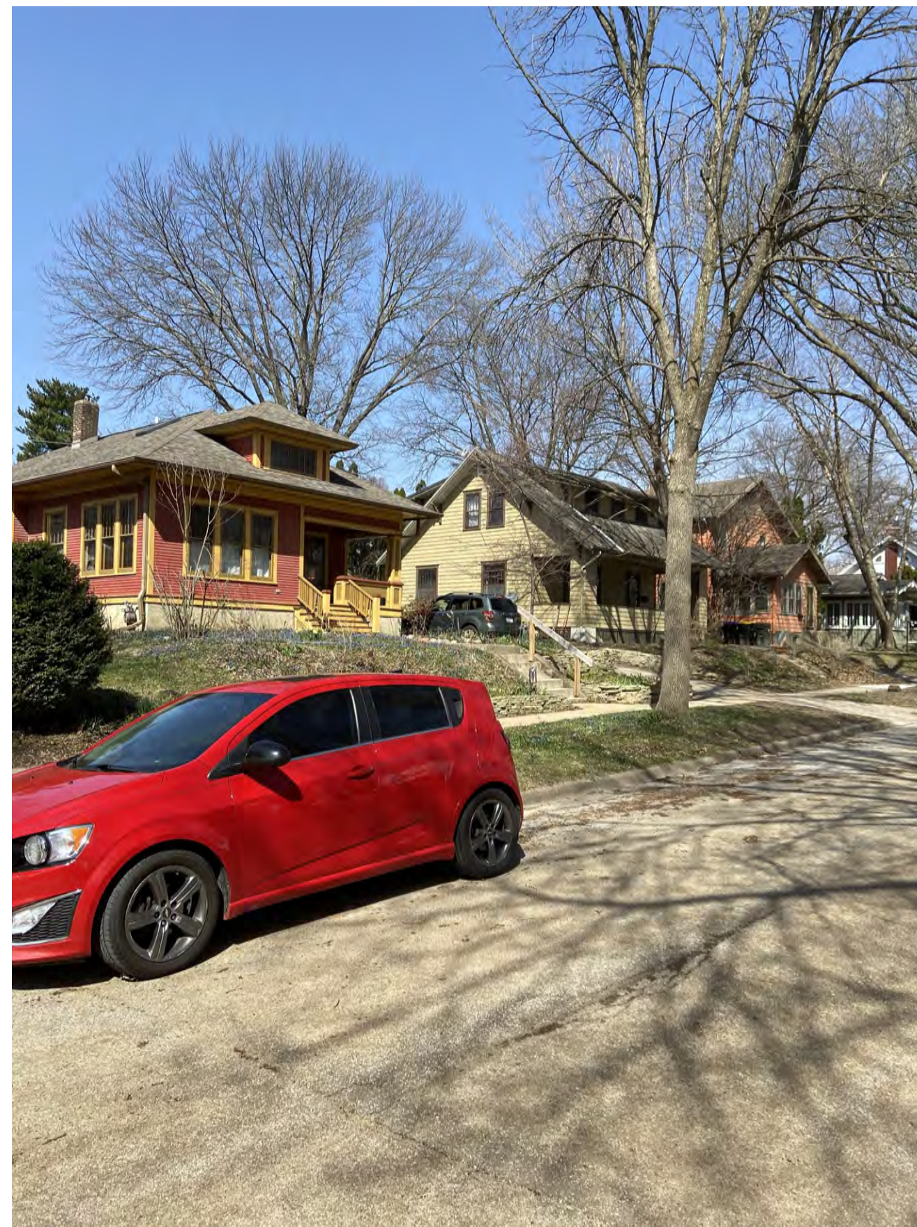
EXISTING PRIMARY FACADE PHOTO
