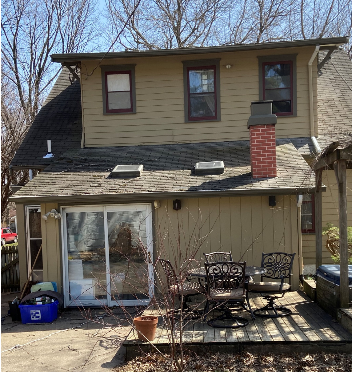
Existing one-story rear addition to be removed (dormer above to remain)
