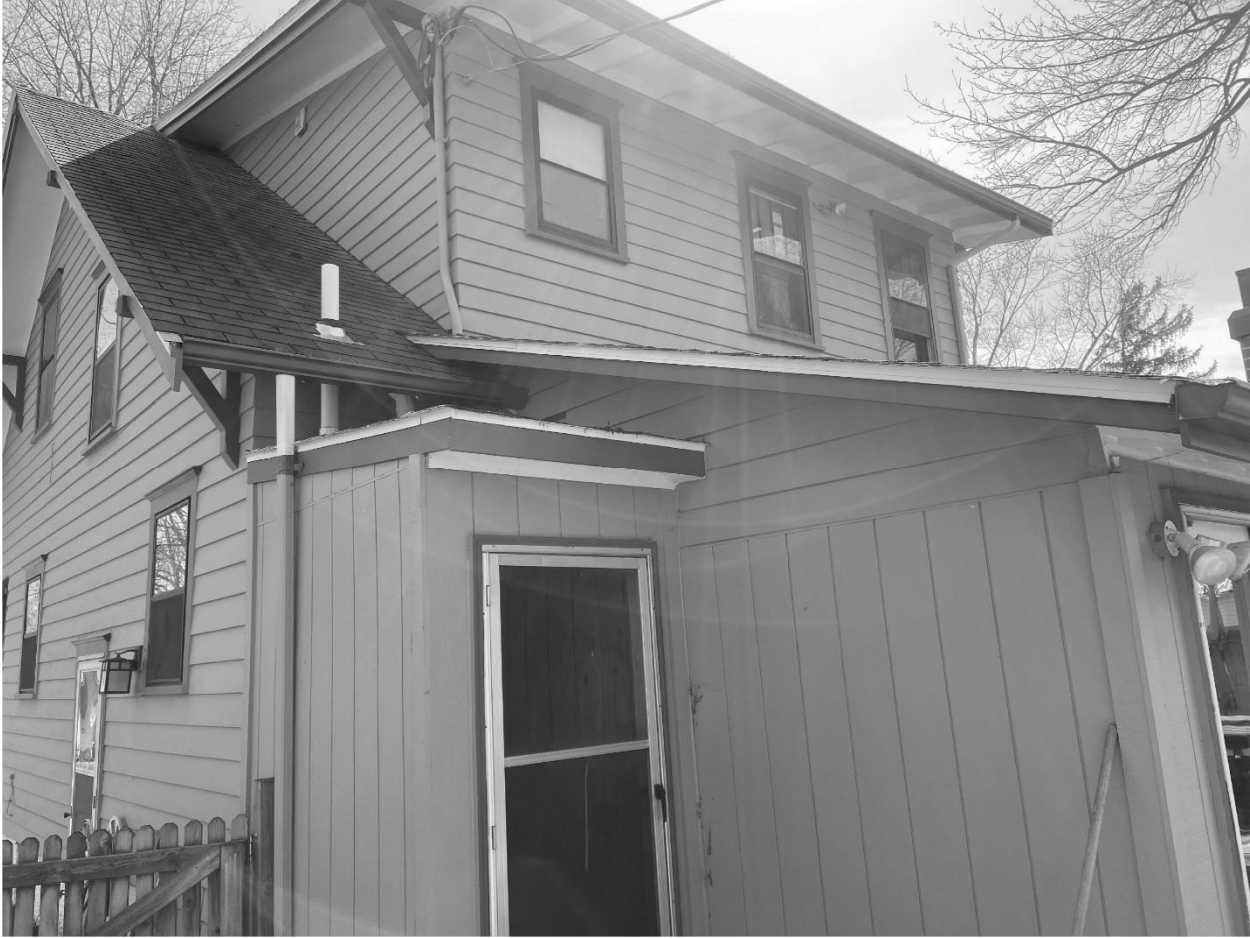
Photo showing rear existing rear addition, entry enclosure, and dormer (to remain)
