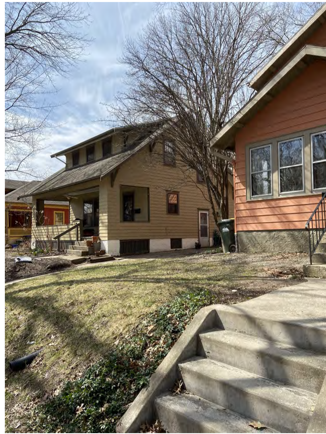
EXISTING PRIMARY FACADE PHOTO
