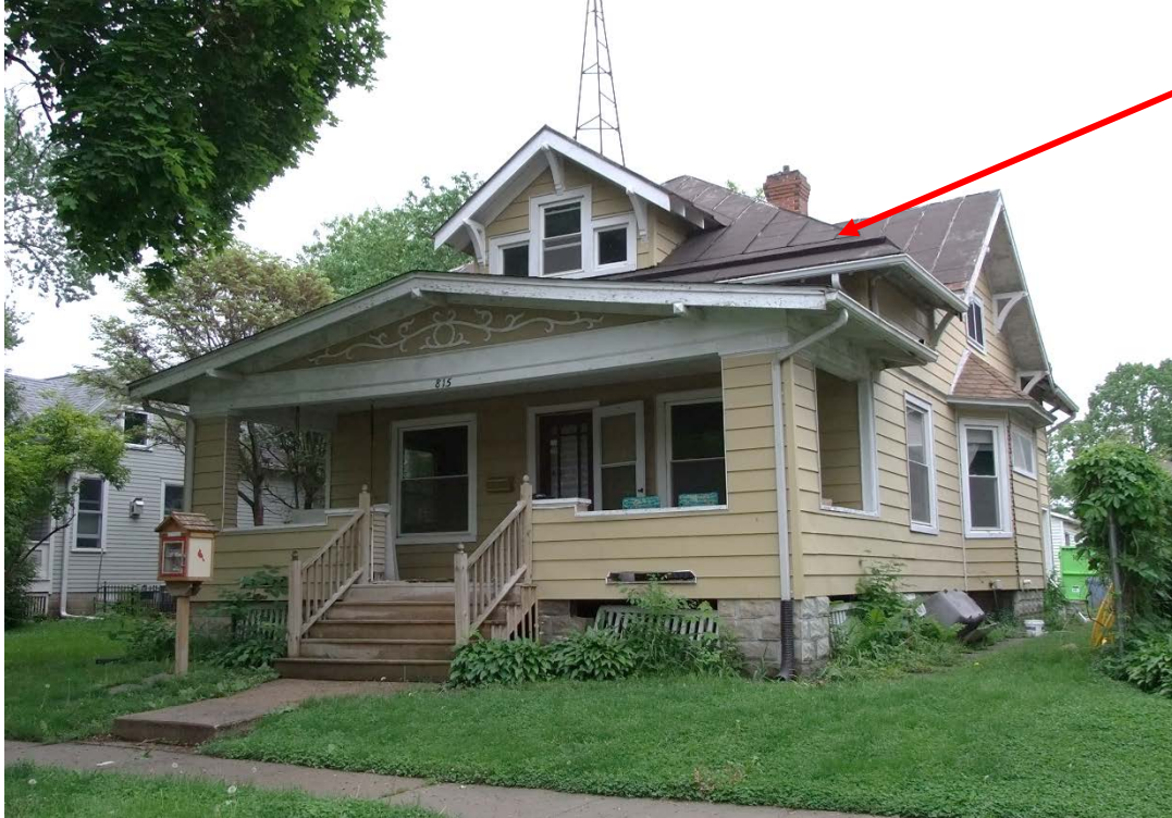
815 Bloomington Street – internal gutter marked
